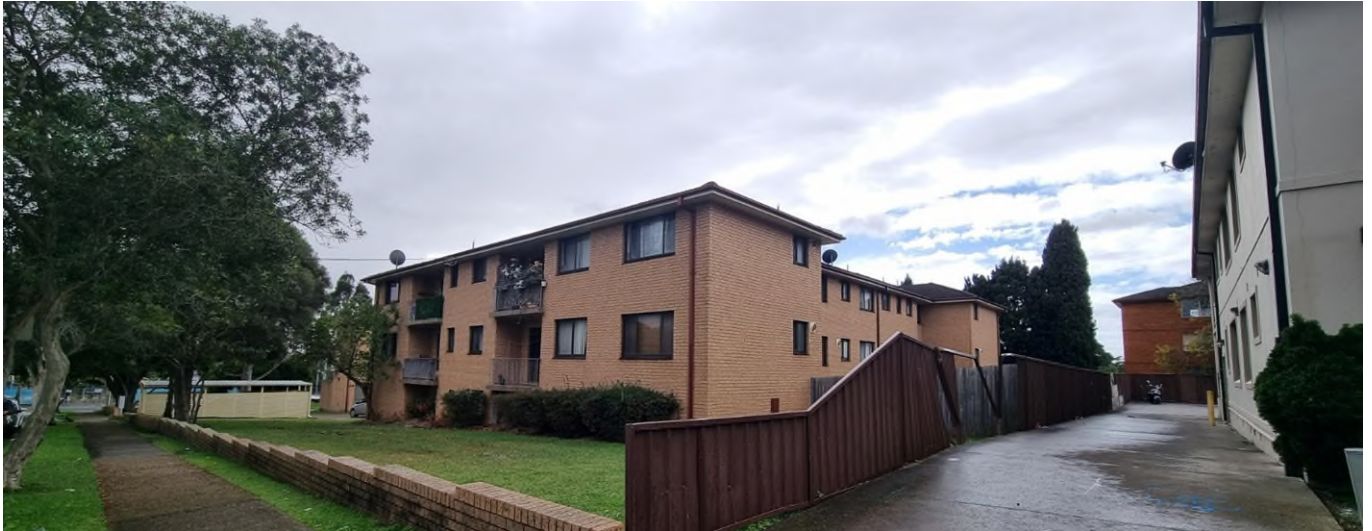
Figure 3 Development site view from Dudley Street – 150-152 The Boulevard, Punchbowl (Source – Homes NSW, 20 May 2025).
