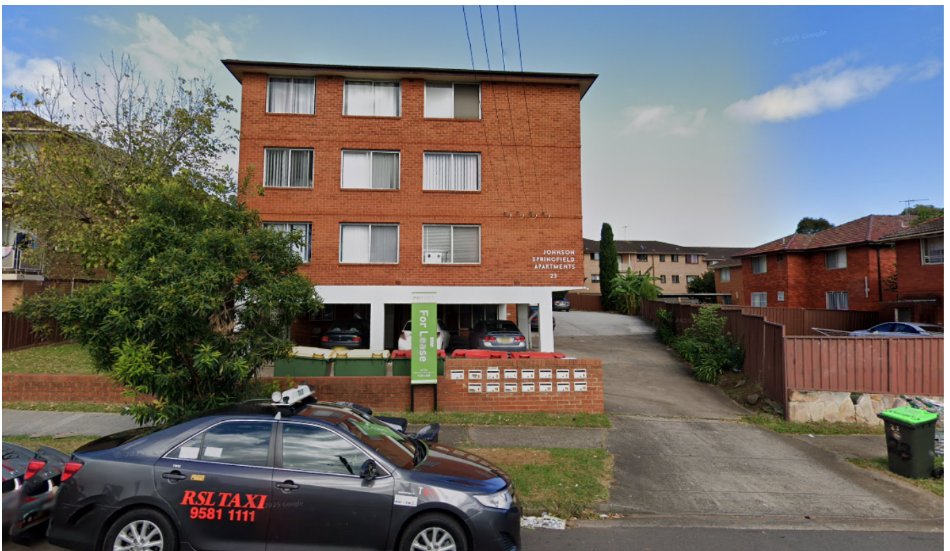
Figure 6 Adjoining development - 27 Rosemont Street (Source - Google Streetview obtained on 26 May 2025)
