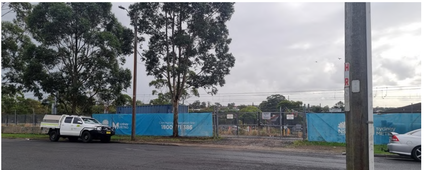
Figure 8 Existing rail infrastructure located opposite the site to the north along The Boulevard, Punchbowl (Source – Homes NSW, 20 May 2025).
