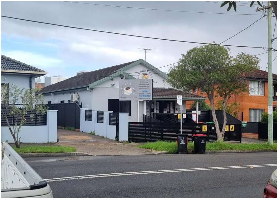
Figure 11 Adjacent property at 21 Dudley Street southwest of the site (Source – Homes NSW, 20 May 2025).
